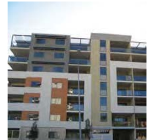
External Facade Walls
