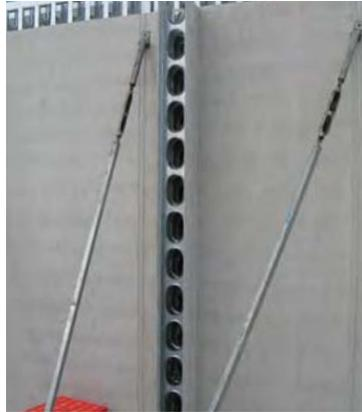
The initial joint connecting the 'T' wall to the AFS Logicwall® track on the through wall should be glued and screwed.
