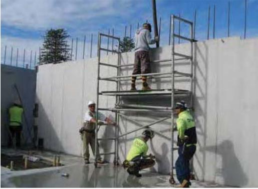
Consideration should also be given to the positioning of braces to provide the best results and also to minimise restriction of free movement by personnel around the site. If the walls are going to need to be filled off a mobile scaffold, it is preferable to run the braces in a way that leaves one face of each wall clear.
