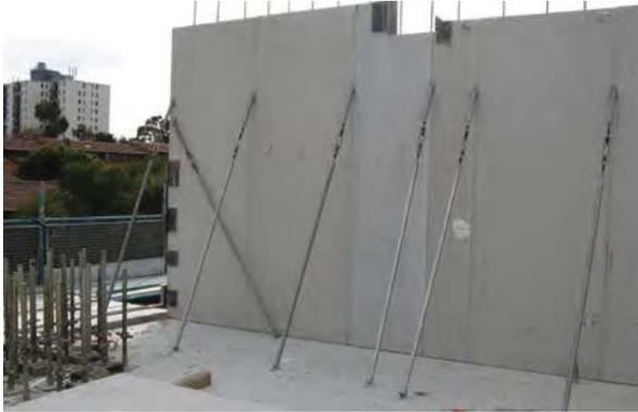
positions to push/pull the panel into alignment. AFS Logicwall® needs to be installed to achieve a tolerance of +/- 4mm over any 1800mm plane. In the case of corners it is not uncommon to use 3 or 4 braces.
