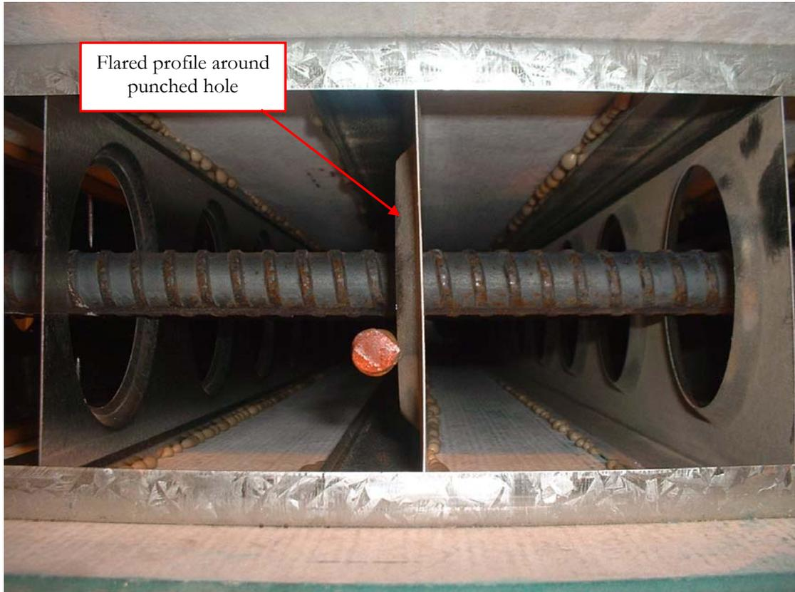
Figure 2 *Flared profile in the steel stud*
