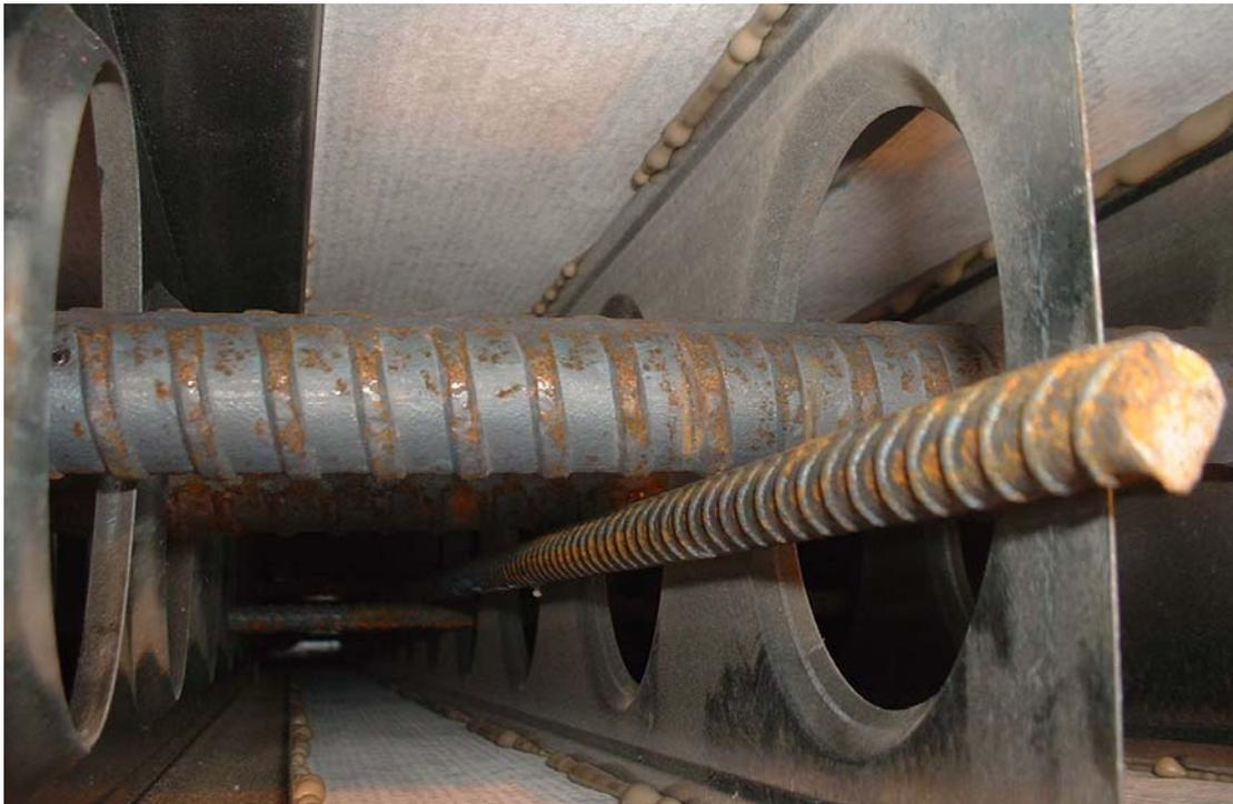
Figure 4 *Vertical Reinforcing bar being held central in wall width by the horizontal reinforcing*
