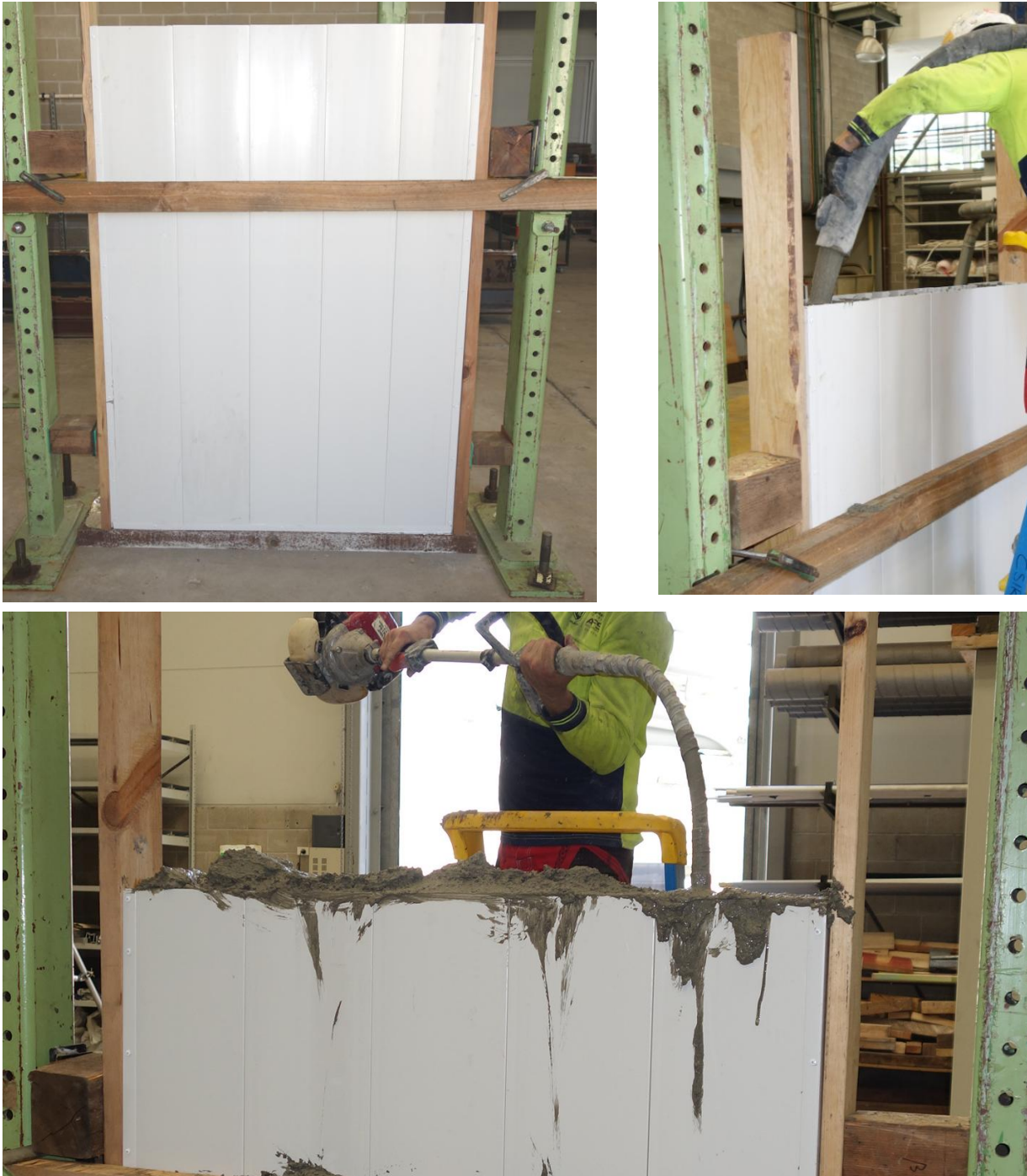
Figure 2 Preparation of wall panel for water penetration and leakage test
