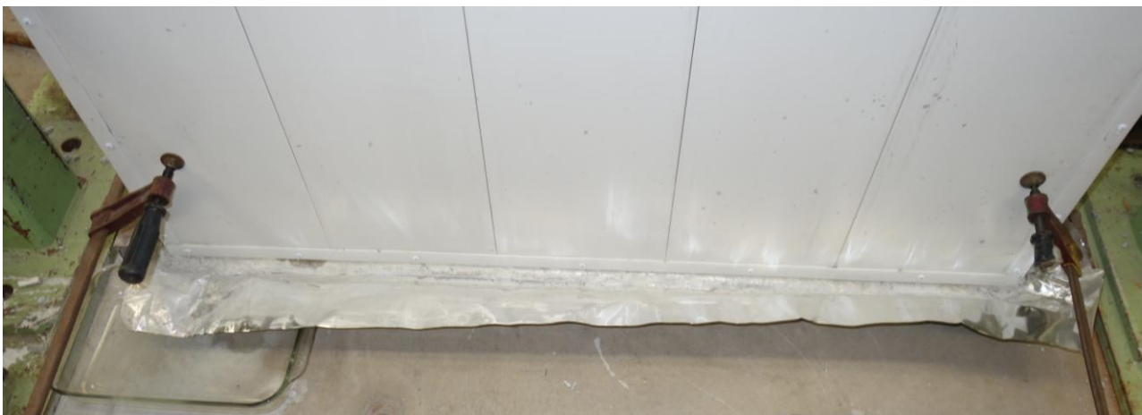
Figure 5 Flashing located at the base of the Wall panel
