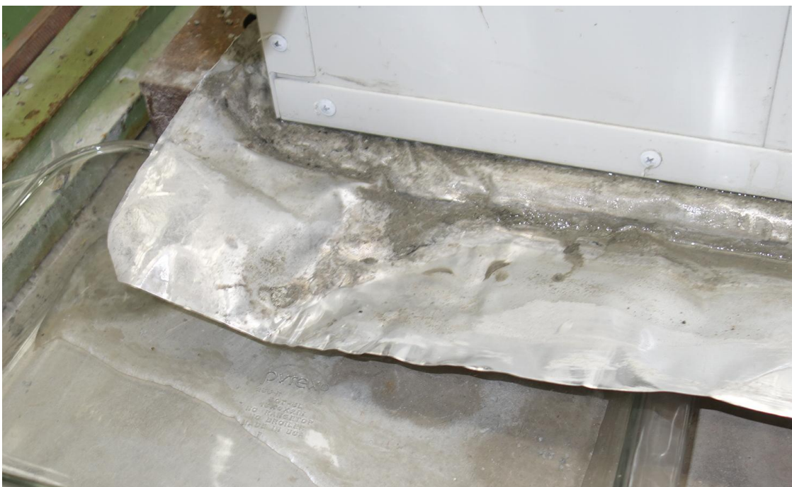
Figure 9 Observation for water penetration at wall panel's base (end stop)
