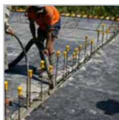
6. Concrete Core Filling
